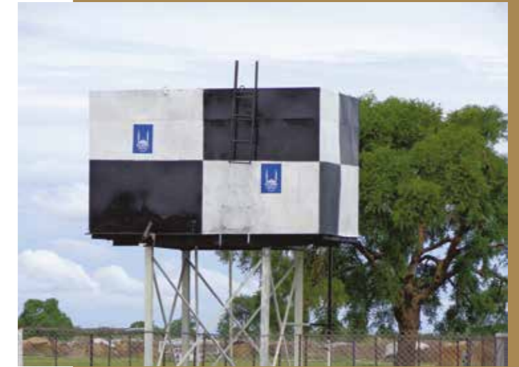
Above: Rehabilitated water yard.
