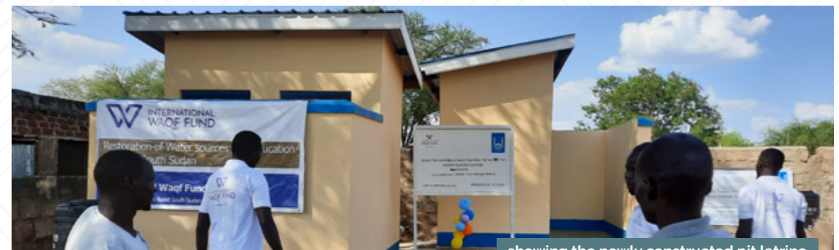
showing the newly constructed pit latrine
